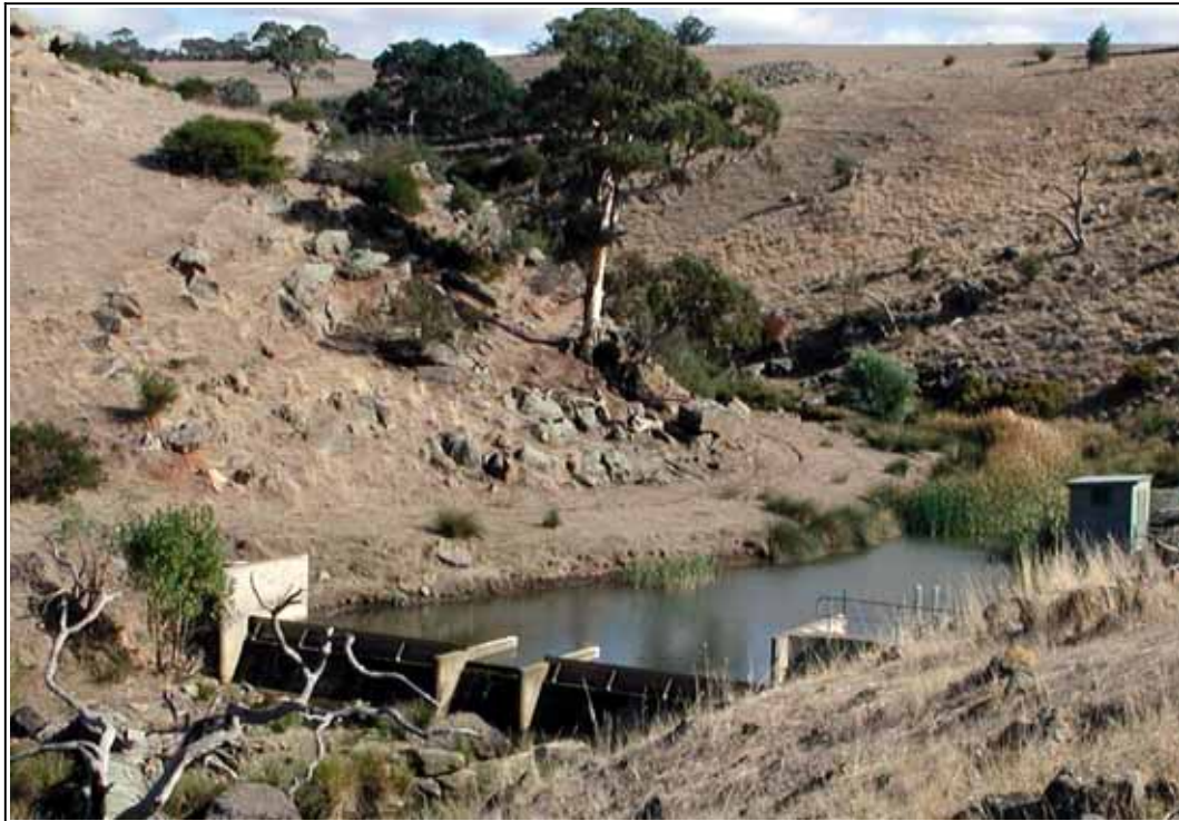
Figure 5. Streamflow gauging station AW426503 (Angas River @ Angas Weir)
