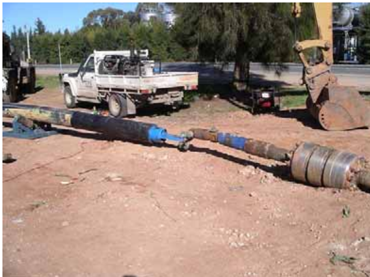
Figure 16. Commencement of pullback
