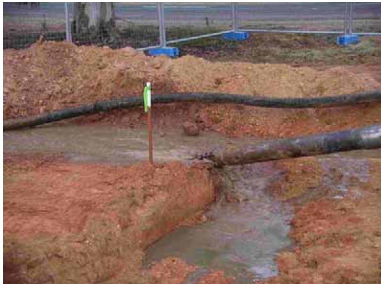
Figure 13. Commencement of pilot drill hole with blade bit
