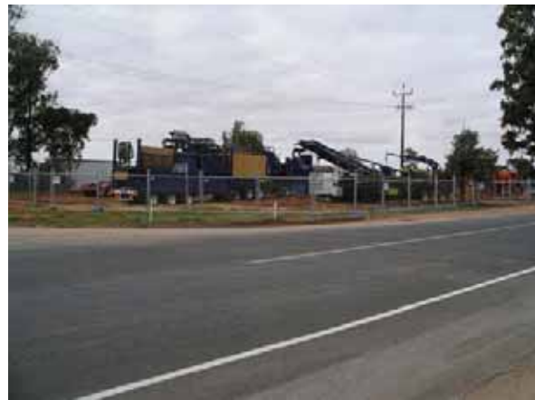
Figure C2. Site safety fencing
