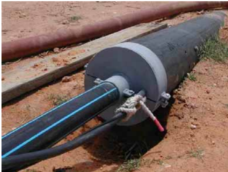
Figure 18. Outer product pipe fitted with steel end cap
