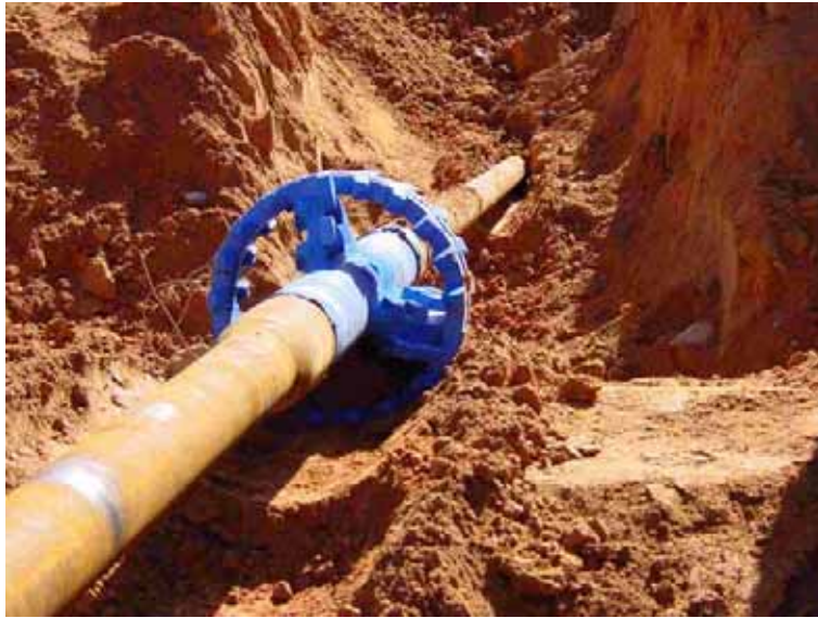
Figure 15. Commencement of reaming
