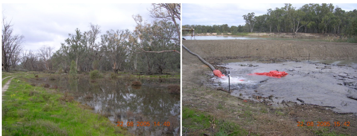
Figure 4. The left image is of the floodplain depression filling with water. The right image is of water being pumped from the river into the depression over the constructed earth bank.
