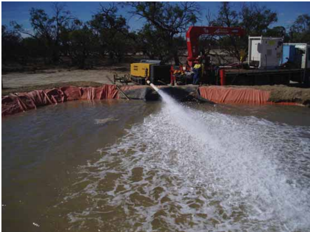
Figure 6. Airlifting looking east
