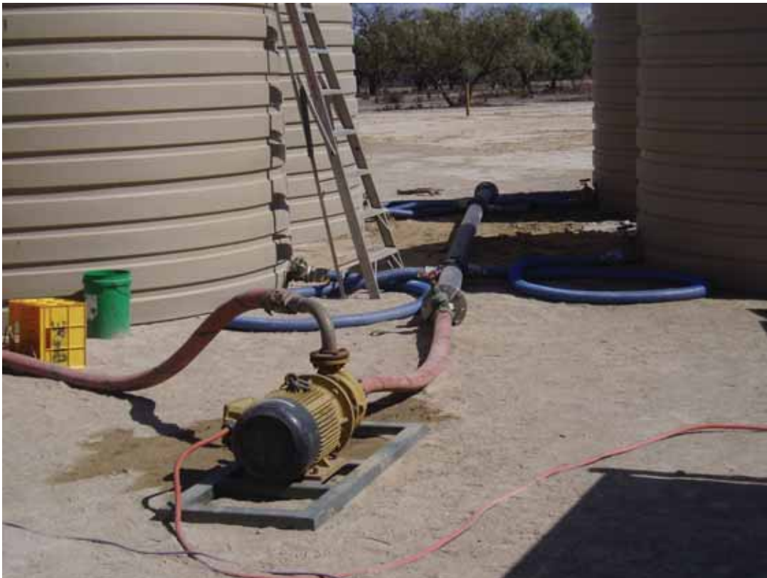
Figure 13. Network of pipes connecting the holding tanks to the pump
