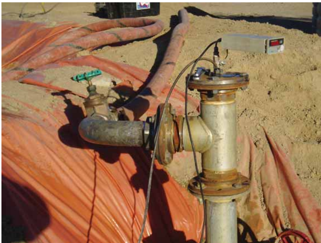
Figure 14. Well headworks
