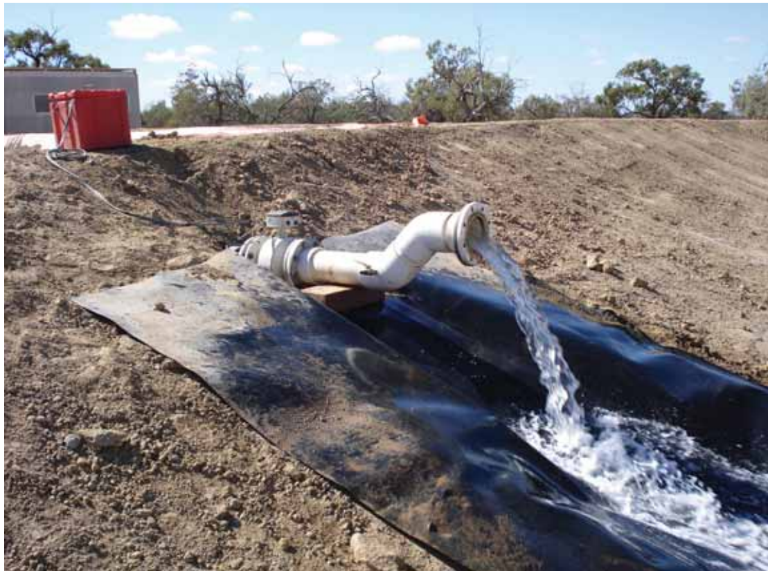
Figure 4. 150 mm PVC pipe connecting the dams with attached flow meter
