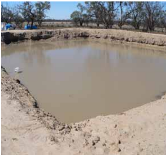
Figures 5, 6. Unlined holding dam and disposal sump (mud pit). The holding dam was used to store water during the mixing of drilling fluid; and to store water that was produced during development. The disposal sump collected unused sample cuttings as they passed over the shale shaker. The de-sander in the (top/middle) was used to separate the very fine material suspended in the drilling fluid that passed through the screen of the shale shaker (Photos courtesy Tony Herbert).
