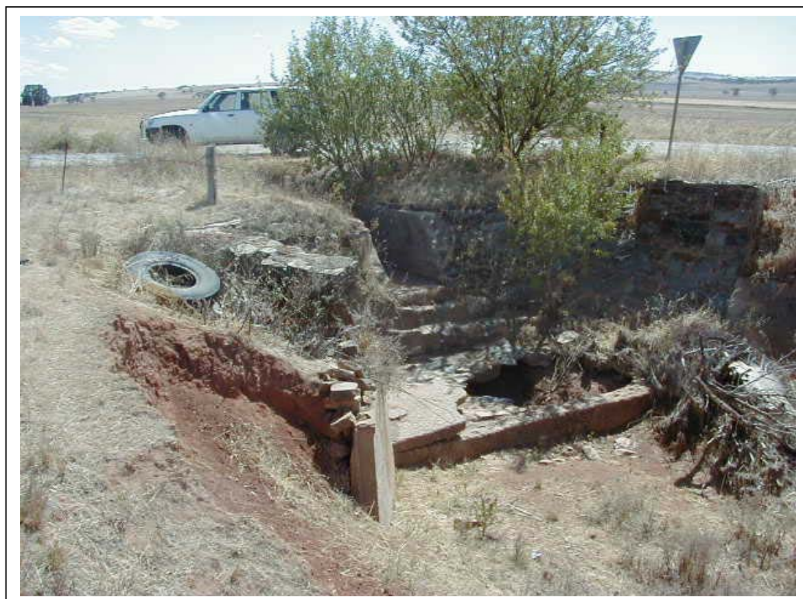
Plate 7.8 Culvert in the Mid Light subcatchment undermined by erosion processes
