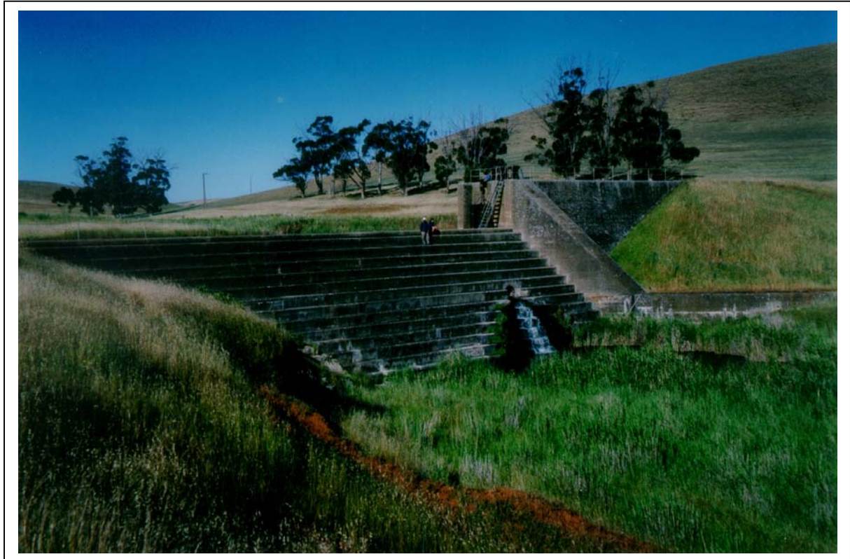
Plate 7.12 Bundaleer weir in the Bundaleer and Freshwater subcatchment: the bed level above the weir is significantly higher than below because of the amount of sediment transported from upstream and trapped by the weir. The weir is a significant barrier to fish migration.
