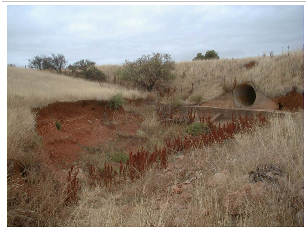
Plate 7.9 An undercapacity culvert that has caused downstream erosion and scouring in the Upper Rocky subcatchment
