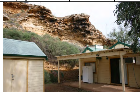
Limestone cliff overhang with tension cracks.
