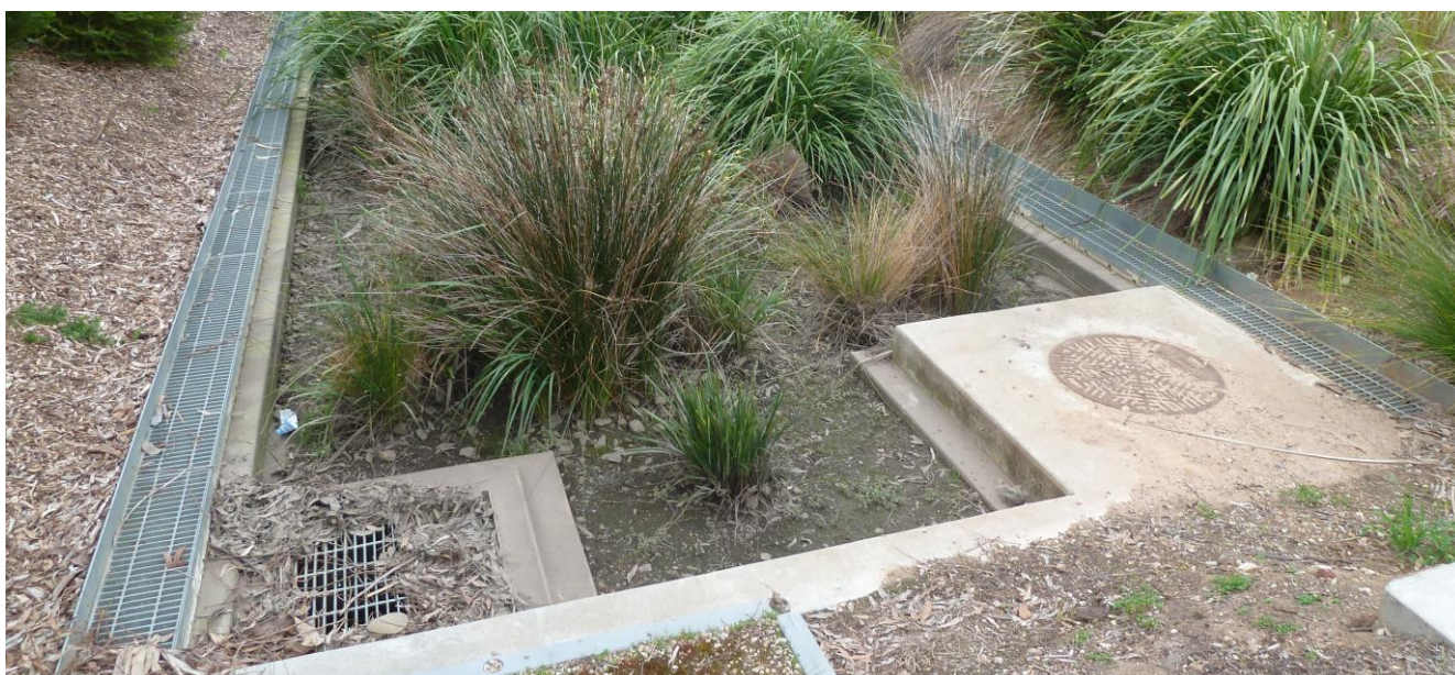
Figure 3-2. Lochiel Park MAR scheme: The vertical infiltration beds look similar to a standard garden bed (top), but a closer inspection reveals their purpose (bottom).
