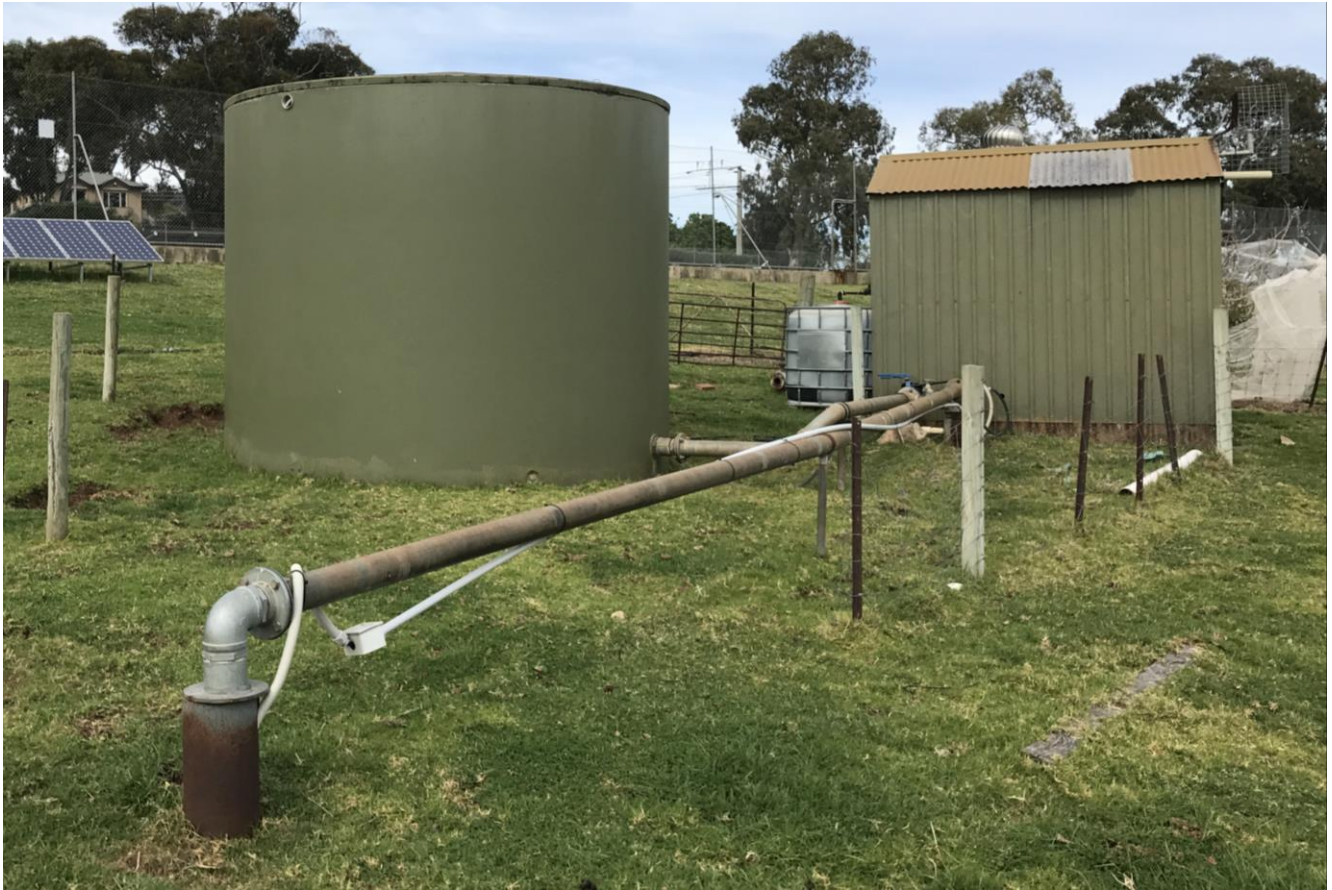
Figure 3-1. Scotch College MAR scheme: The injection well is next to the shed, and extraction well in the foreground.
