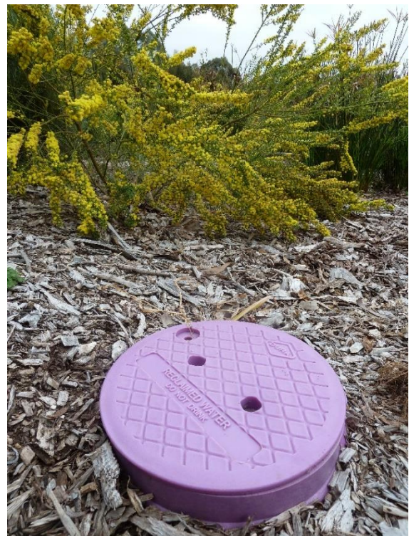
Figure 4-1. Alternative water supplies, indicated by purple pipes and fittings, irrigate many public reserves and gardens
