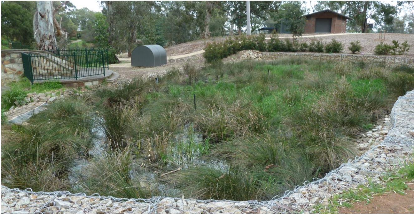
Figure 3-3. Ridge Park vertical biofiltration bed: Water is pumped from the creek and is filtered as it percolates through the wetland bed. An injection well is contained in the grey-domed box.
