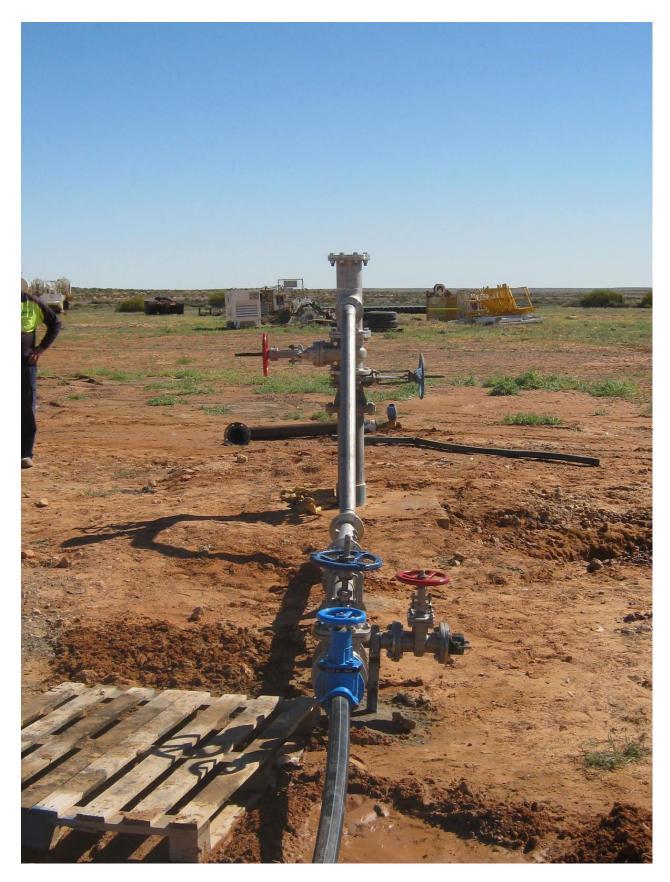
Figure 9. Headworks of Mulka Bore No. 2
