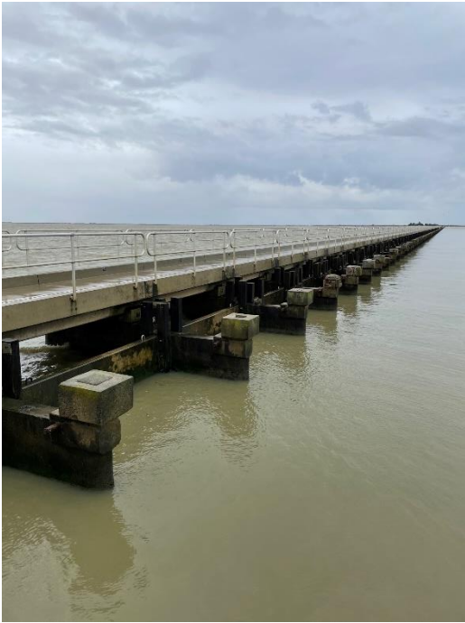
Tauwitchere barrage on a stormy day last week (K. Williamson, DEW)
