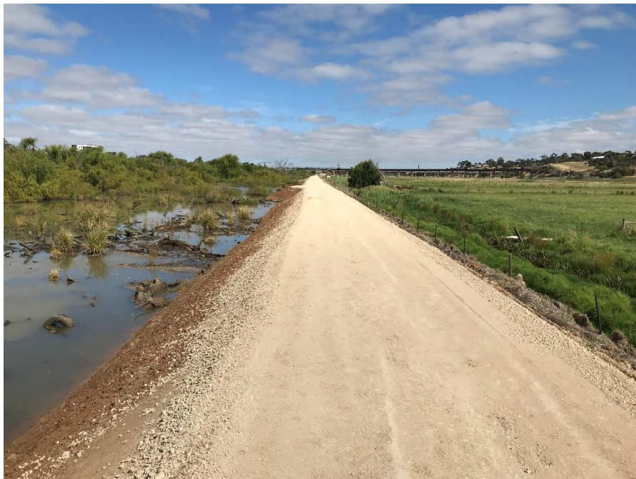
Figure 1: Recently repaired Burdett levee bank downstream of Murray Bridge (DEW)
