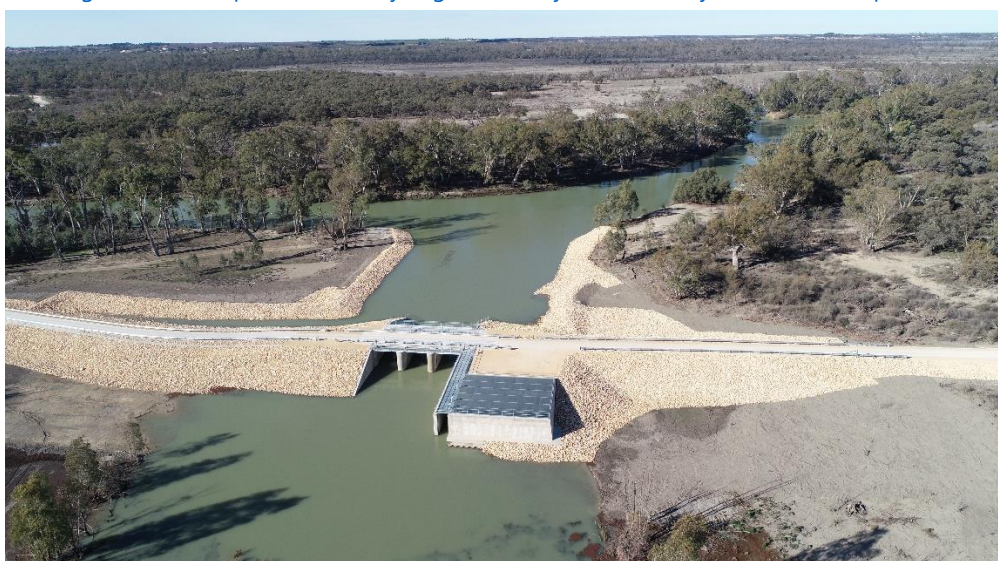
Figure 1: The Splash regulator on the Katarapko Floodplain at the beginning of the 2020 watering event (Daniel Haines, SA Water)
