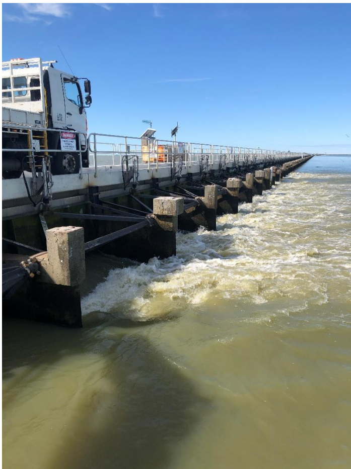
Figure 2: Water being released to the Coorong through barrage gates at Tauwitchere barrage (Photo: Kimberley Williamson)
