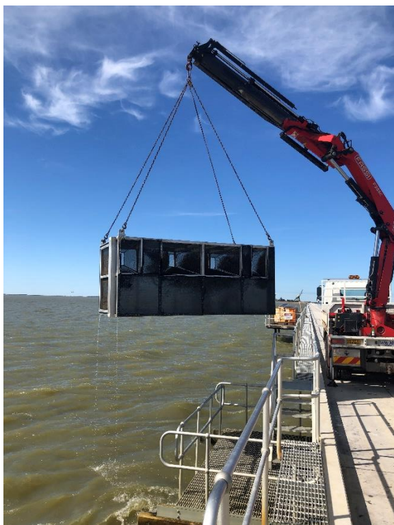
Figure 1: Fishway trap being pulled from the trapezoidal fishway at Tauwitchere barrage for fishway monitoring in August 2020 (Lake Alexandrina side of the barrage) (Photo: Kimberley Williamson)
