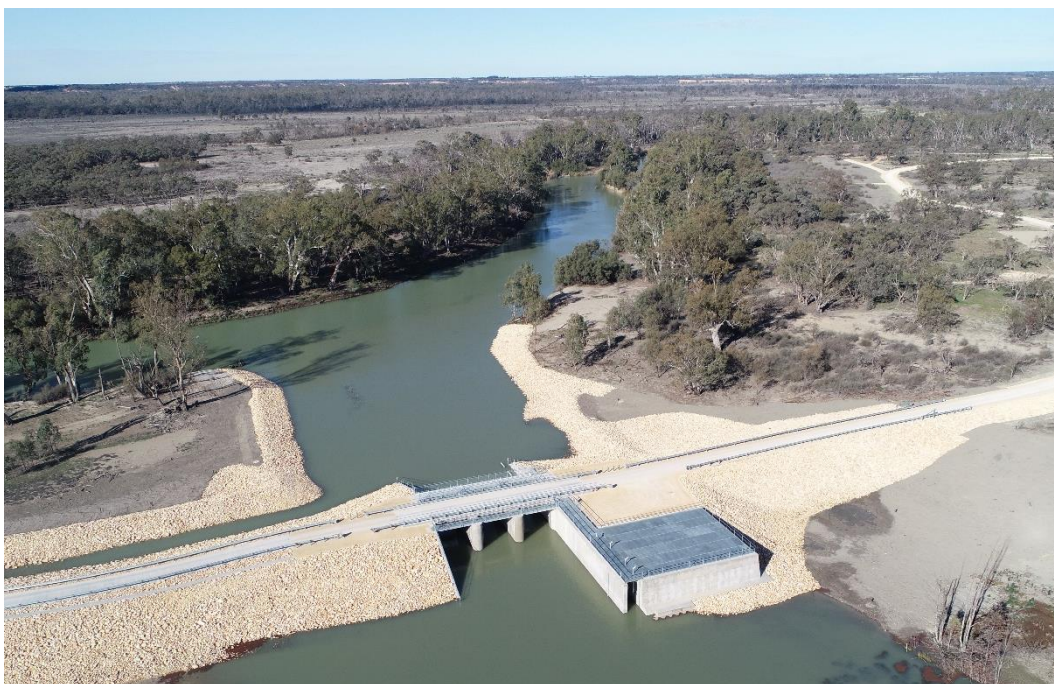
Figure 2: main environmental regulator on the Katarapko Floodplain known as 'The Splash' (Source: Dan Haines, SA Water)
