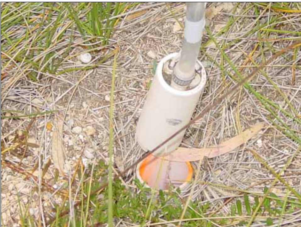
Plate 4. Piezometer RIL013 with 12V submersible Whale® pump.
