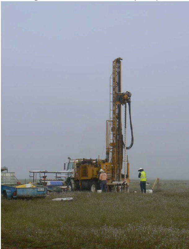
Figure 21. Drilling at RS006A01, November 2007
